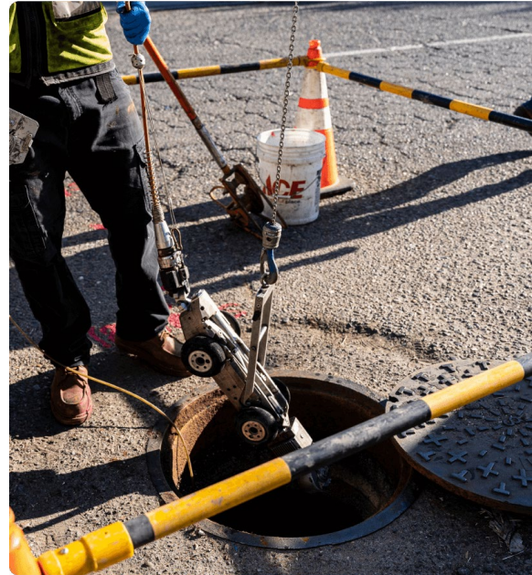
Figure 4. APS Deploying a CCTV Rover
