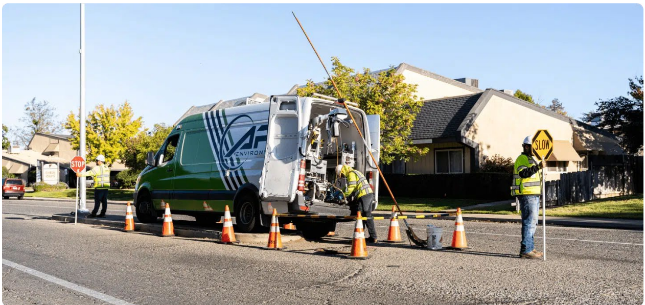
Figure 2. APS Inspecting a Sewer in a Residential Neighborhood
