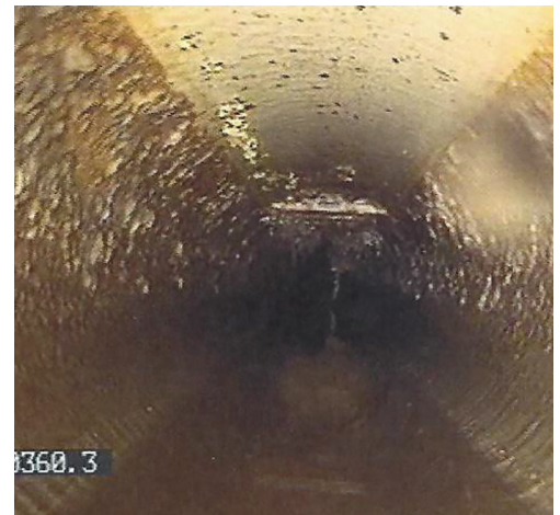
Microbe-Lift was used to treat 10-inch sewer line with recurring heavy grease buildup. Before and after photos show level of FOG reduction after five months of once a week treatment in a manhole 500 feet upstream.
