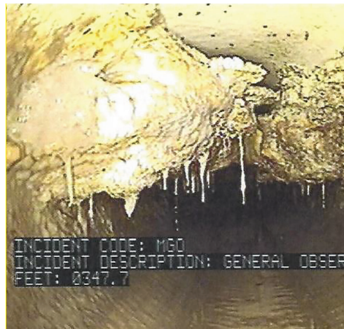
Microbe-Lift was used to treat 10-inch sewer line with recurring heavy grease buildup. Before and after photos show level of FOG reduction after five months of once a week treatment in a manhole 500 feet upstream.
